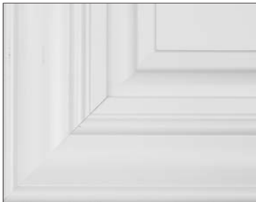
Example of front joint separation
